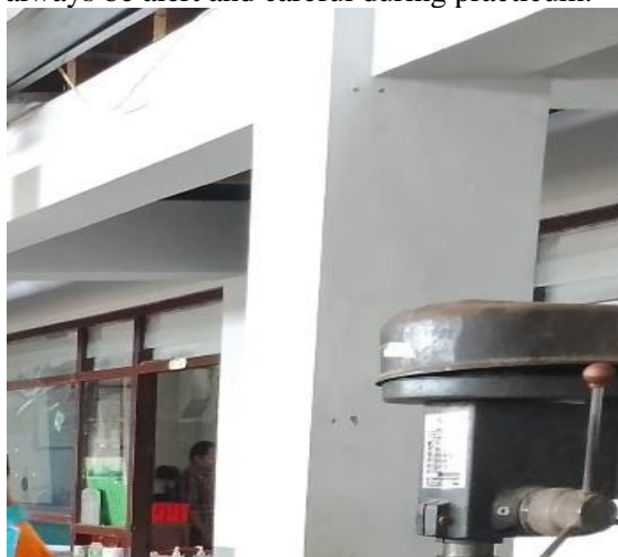
Figure 6. Unavailability of Work Safety Warning Signs
