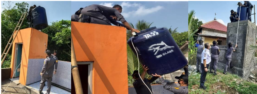
Gambar 8. Proses instalasi reservoir
