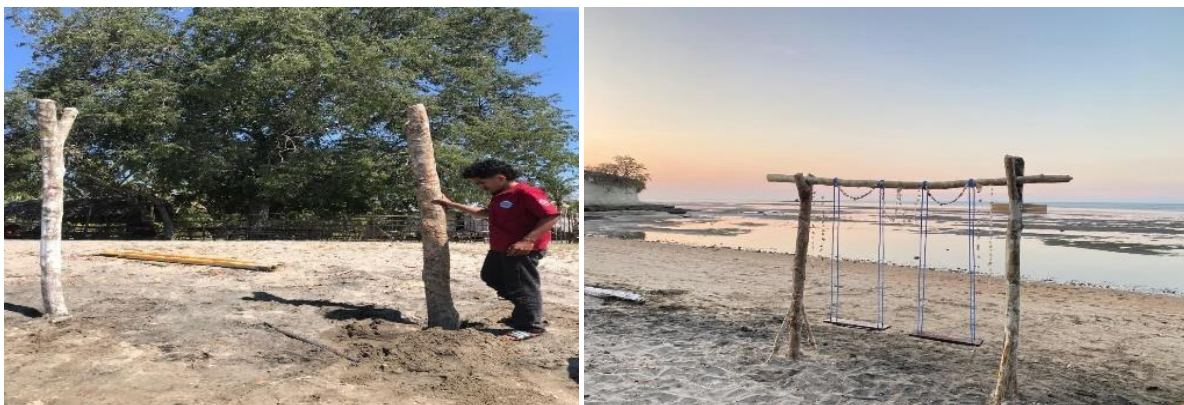
Figure 2 . Installation of seaside swing
