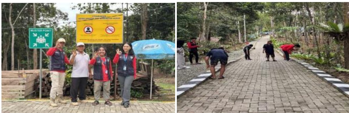
Figure 2. The installation of environmental damage prohibition and occupational safety signage, along with the painting of tracking path markings along the roadside at the Meranti Forest Tourism location.
